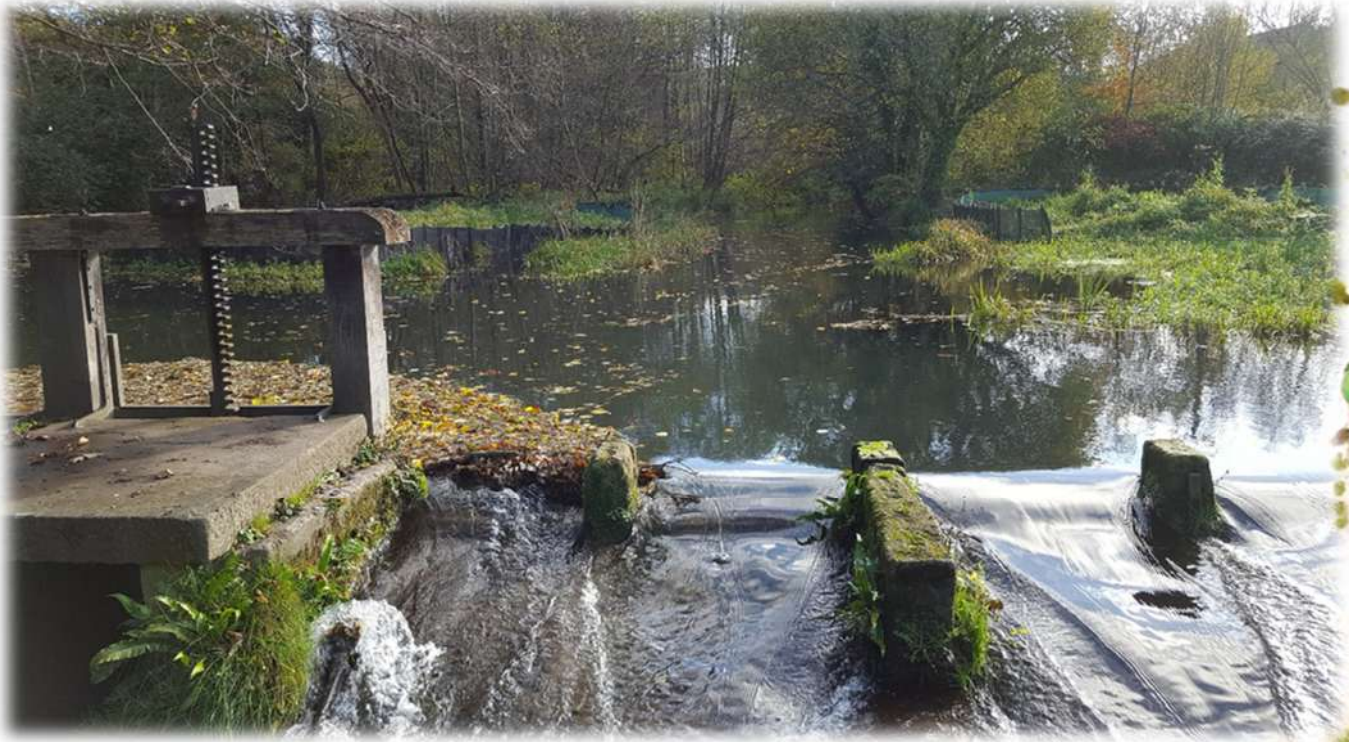
The sluice gate and spillway at Arundel Mill Pond today
